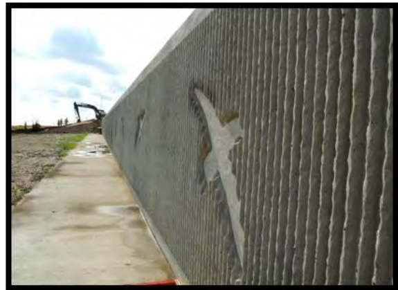
Photograph 4-5. Aesthetic concrete stamping for floodwalls at the Williams Boat Launch.
