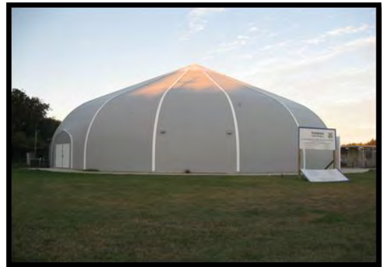
Photograph 4-11. Phoenix High School Gym enclosure.
