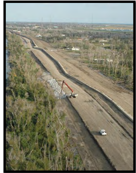
Buras floodwall construction
