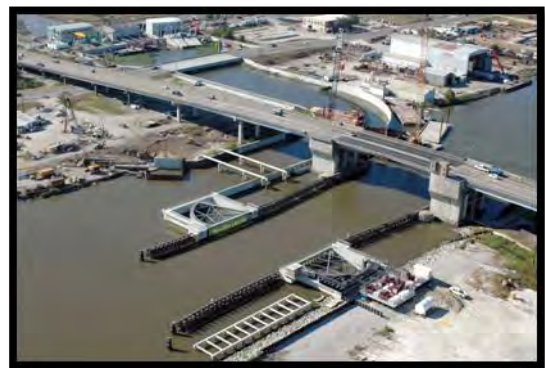
Photograph 2-2. Harvey Canal sector gate.
