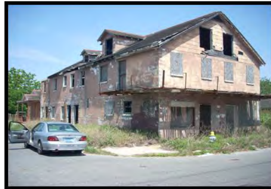
Photograph 4-17. Abandoned structure in the Lower Ninth Ward.
