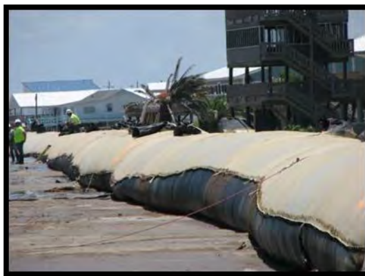
Initial placement of geo-textile tubes
