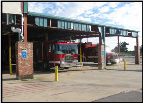
Photograph 4-19. Buras Volunteer Fire Department temporary headquarters.
