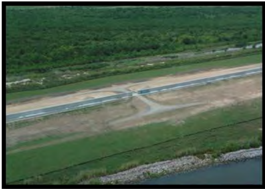
Photograph 4-2. Wildlife opening in the Chalmette Loop Levee T-wall
