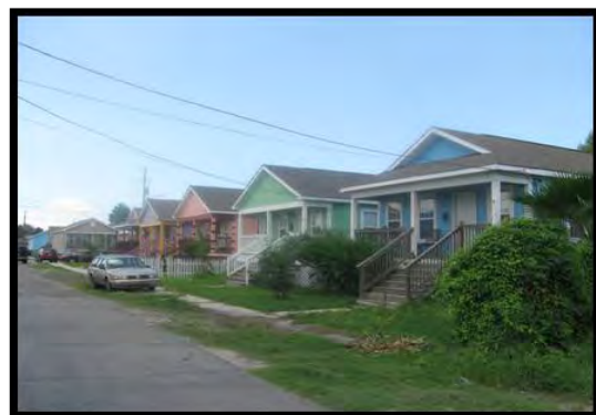
Photograph 4-15. Rebuilt residences in the Lower Ninth Ward.
