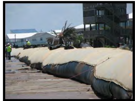
Photograph 3-2. Initial placement of geo-textile tubes.
