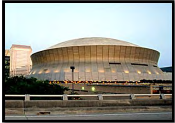
It would take 4.4 million cubic yards of borrow to fill the Mercedes-Benz Superdome, which would need to be filled 21 times to equal the fill needs for the entire HSDRRS.
