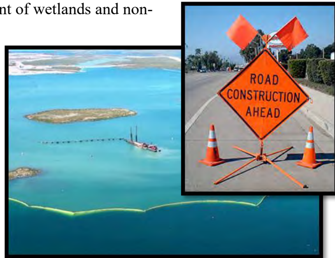
Examples of signage and silt curtain mitigation measures
