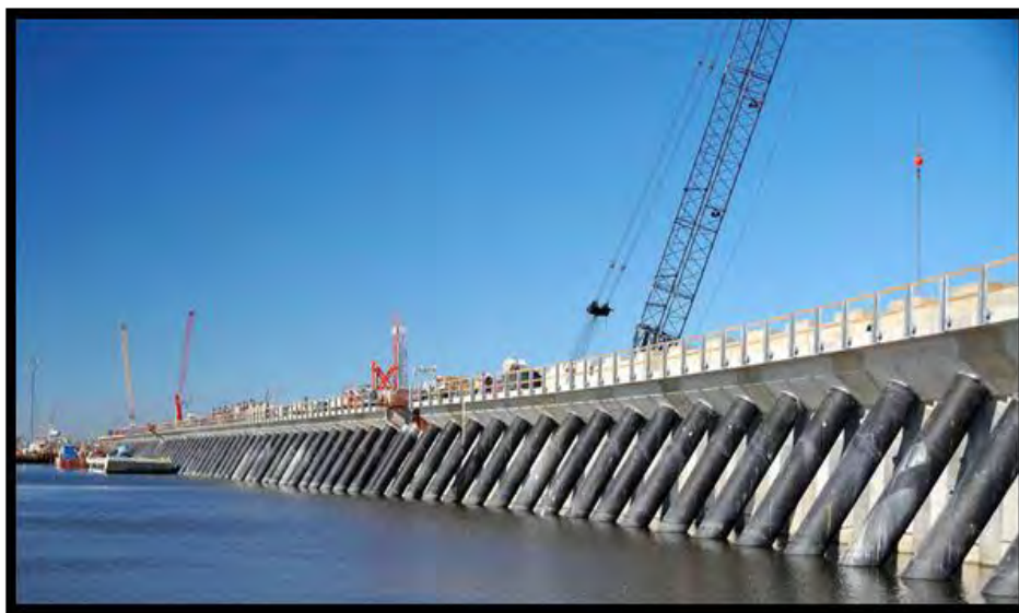
Photograph 2-1. IER #11 HSDRRS Borgne barrier under construction.
