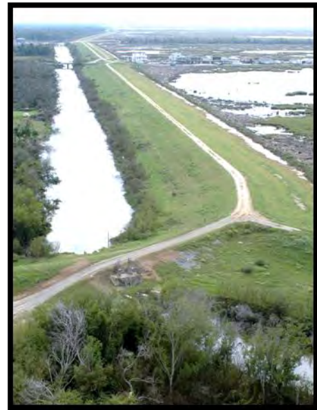
Earthen levee with access road near St. Jude
