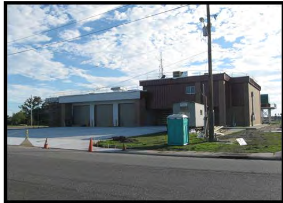
Photograph 4-20. New headquarters for Buras Fire Department.
