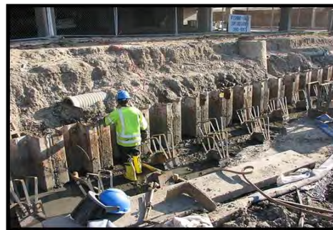
HSDRRS sheet pile construction activities
