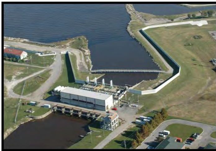
Duncan Pump Station
