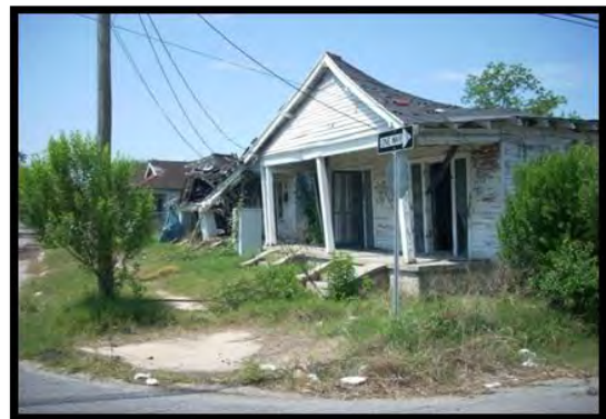
Photograph 4-13. Damaged properties due to Hurricane Katrina.
