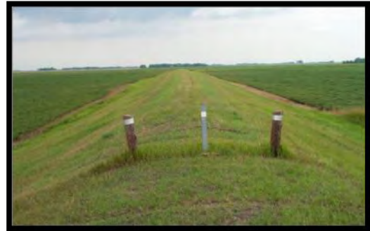
Example of an earthen levee in southeast Louisiana
