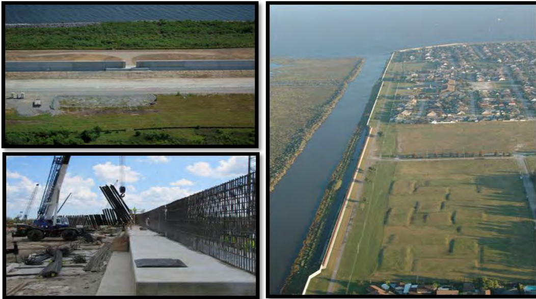
Photograph 4-4. Examples of floodwalls and levees with floodwall caps.
