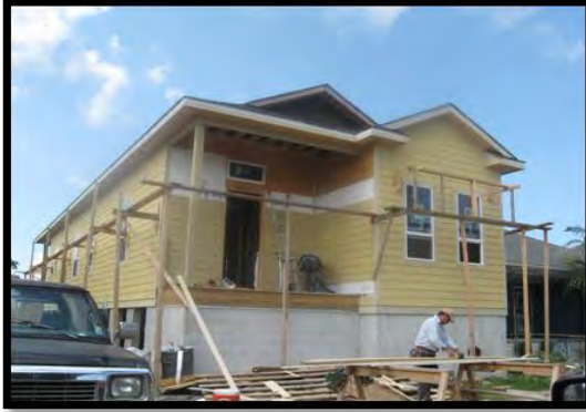
Photograph 4-16. Housing reconstruction in the New Orleans Lakeview area.
