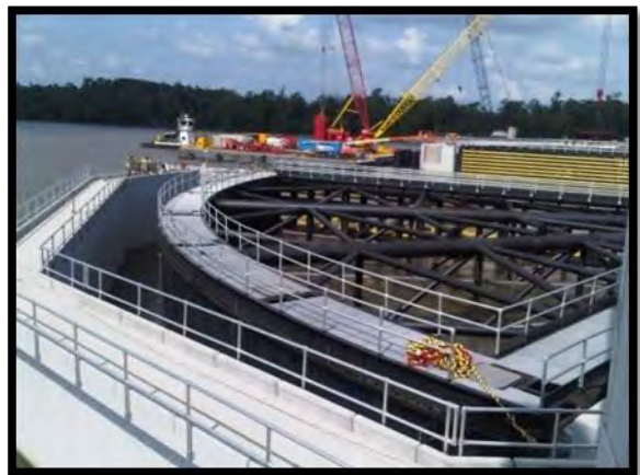
Example of HSDRRS sector gate
