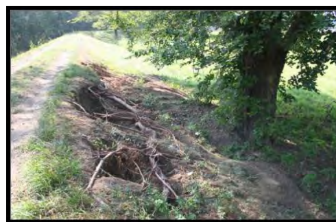
Photograph 4-1. Impacts on an earthen levee from tree roots.
