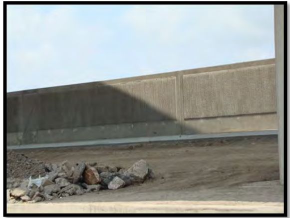
Photograph 4-6. Aesthetic articulated fin finish for floodwalls at the Franklin Ramp.
