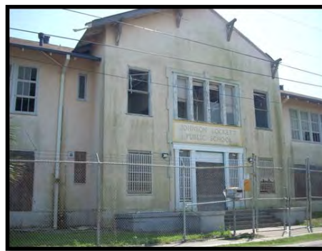
Photograph 4-10. Condemned school in Orleans Parish.
