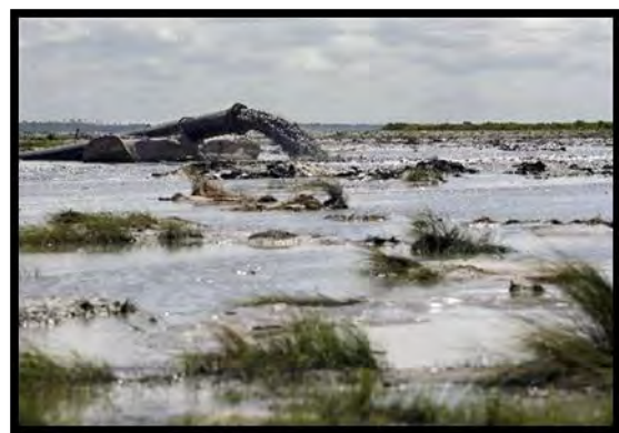
Wetland restoration technique: beneficial use of dredged material
