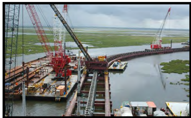
HSDRRS construction of the Borgne barrier
