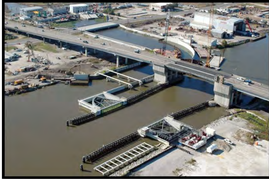
Photograph 8-2. Harvey Canal Sector Gate.
